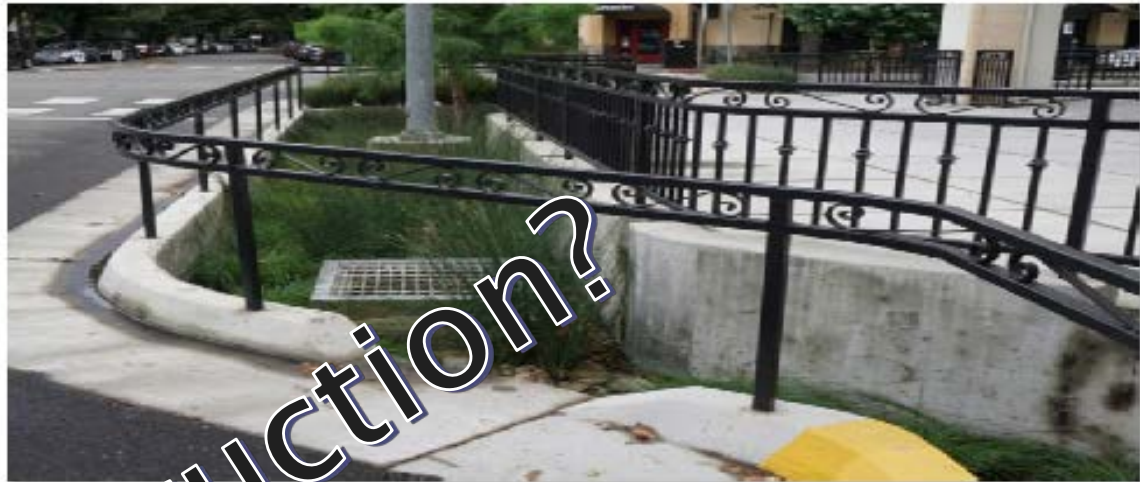
Figure A: Photograph of an Urban Infiltration Trench
