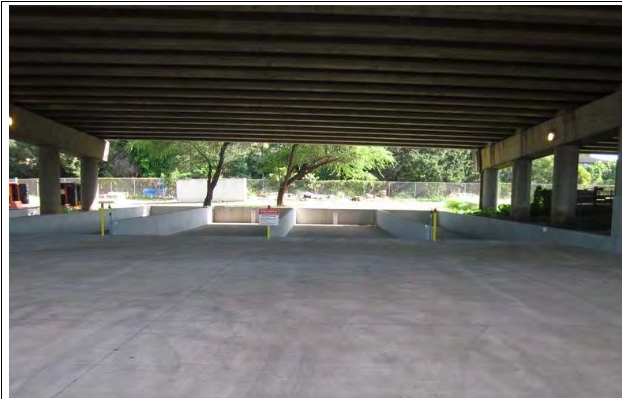
FIGURE 3-7: BASEYARD FUNCTIONAL AREAS – SPECIAL SERVICES SUBUNIT DEWATERING FACILITY
