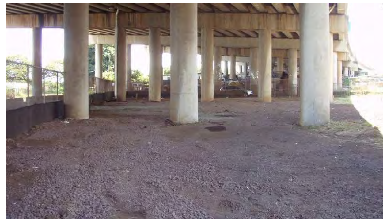
FIGURE 3-1: BASEYARD FUNCTIONAL AREAS – EQUIPMENT SERVICE & REPAIR UNIT SALVAGE EQUIPMENT STORAGE AREA
