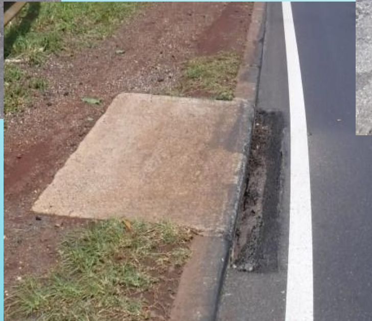
After paving/cut out down to inlet
