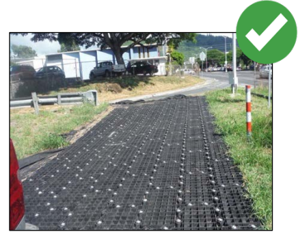
Alternative commercial construction entrance/exit products may be used if approved by the Engineer and installed per manufacturer's specifications.
