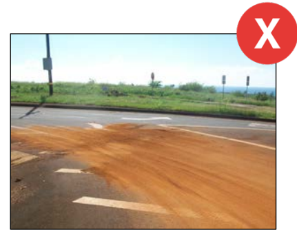
Sediment tracked onto adjacent roadways or paved areas must be removed using dry cleaning methods.
