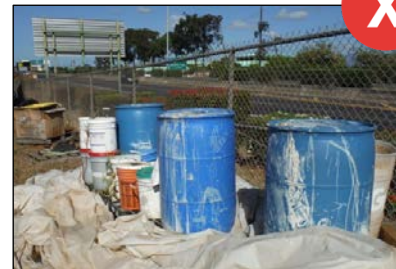
Hazardous materials not stored in a covered facility must be placed in secondary containment and under an impermeable cover.
