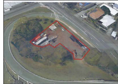
Aerial view of a construction staging area.
