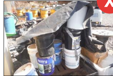
Stacked containers, higher than 2, must be secured from tipping over and under adequate cover.
