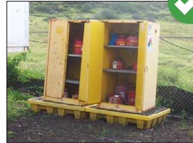
Hazardous materials stored under a covered facility and in secondary containment prevents storm water from coming into contact with materials.
