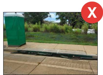
Portable toilets must be located away from drainage systems and waterbodies.
