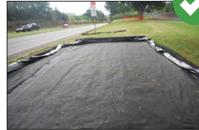
Store vehicles and equipment on a layer of geotextile filter fabric on top of 10 mil plastic sheeting when not being used.
