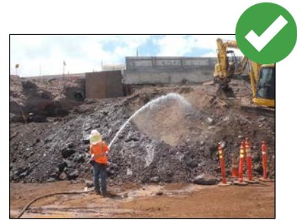
Spraying water on exposed areas and when drilling, sawcutting, jack hammering, or grinding helps mitigate the amount of dust produced on a construction site.
