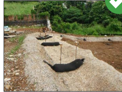
The bottom of the upstream check dam should be at the same elevation as the top of the downstream check dam to promote the formation of small pools between check dams.
