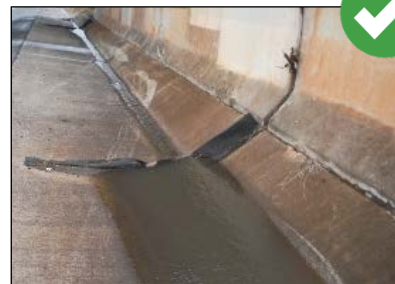
The center of the check dam must be lower than the ends to prevent water from running around the ends and causing additional erosion.
