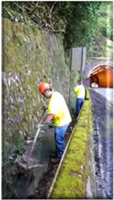
Shovel dirt and debris.
