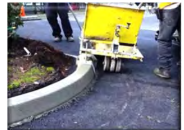
Repairing a curb.
