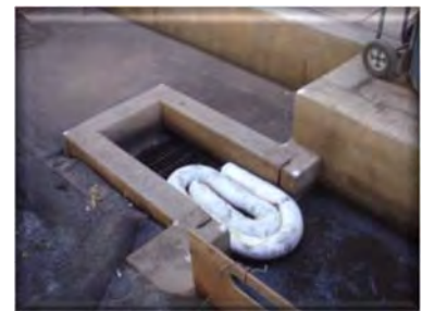
Protect stormwater drains.
