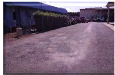
Clean up work site.
