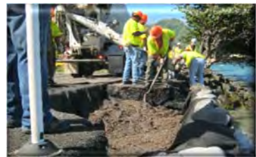
Protect surface water.
