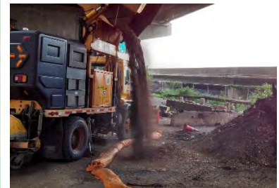
Use berms for stockpiling.
