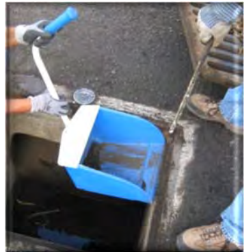
Clean storm drain.
