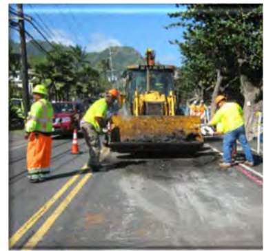
Remove broken asphalt.
