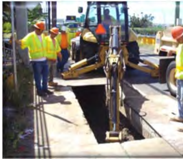
Expose the buried utility.
