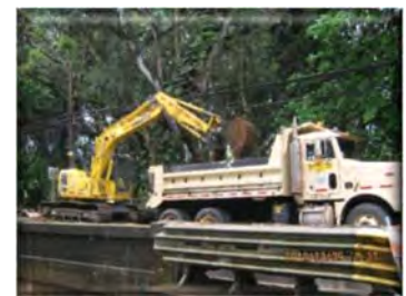
Remove material from work site.
