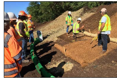
Product demonstrations provide hands-on training opportunities for BMP installation.
