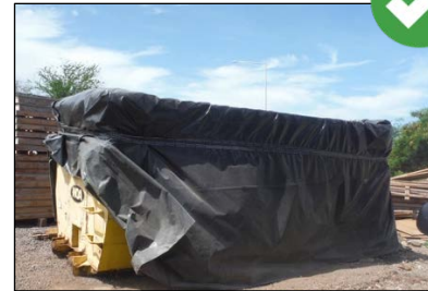
Waste containers must be covered with an impermeable material at the end of the day and when it is not in use.
