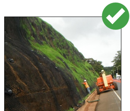
Phase disturbances and use stabilization techniques designed for steep grades if disturbance of steep slopes is unavoidable.
