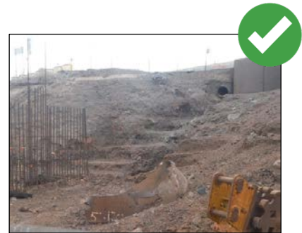
Terracing design and approval must be under the direction of a licensed, qualified engineer.
