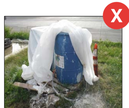
Cleanup procedures must be followed when leaks from vehicles, equipment, and stored materials are evident.
