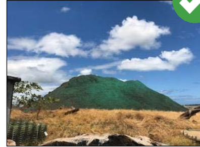
Soil binders can be used on large stockpiles to prevent erosion from wind and rain.
