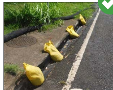
Properly installed curb inlet guards are placed tight to the drain opening and anchored per manufacturer's specifications.
