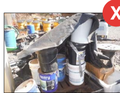
Stacked containers, higher than 2, must be secured from tipping over and under adequate cover.
