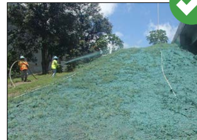
Properly applied hydraulic mulches stabilize disturbed soil by protecting bare soil, increasing infiltration, and decreasing runoff.
