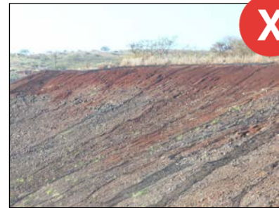
Additional mulch may be needed if erosion of hydroseeded area has occurred.
