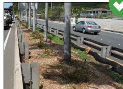
Evenly distribute wood/bark chips on soil surface and maintain a 2-inch mulch depth to tree basins and a 4-inch mulch depth to shrub beds.
