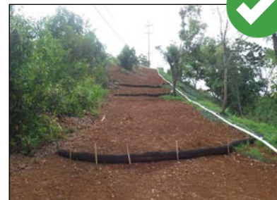
Compost filter berms must be staked into the slope to secure them into the ground.
