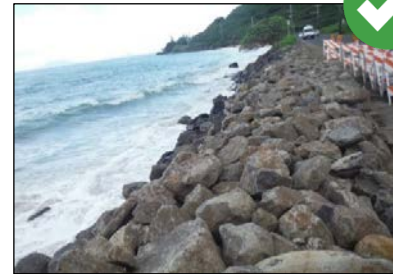
Rip-rap can help prevent or minimize erosion when used to stabilize shorelines.
