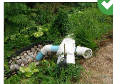
Slope drains may be installed above-ground or buried beneath the slope surface.
