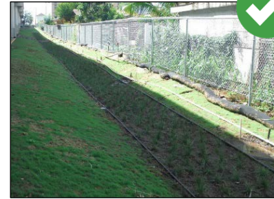
Additional watering or irrigation to supplement rainfall may be needed until vegetation has been established.
