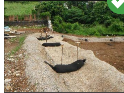
The bottom of the upstream check dam should be at the same elevation as the top of the downstream check dam to promote the formation of small pools between check dams.
