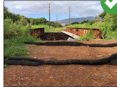
If state waters are located within 50 feet of disturbed area and an undisturbed natural buffer less than 50 feet is used, install double sediment control spaced a minimum of 5 feet apart.
