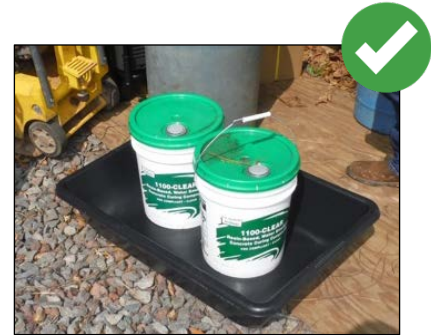
Secondary containment reduces the risk of spills and leaks from getting into storm water runoff, contaminating soil, and injuring workers or visitors.
