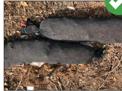
Compost filter socks must be overlapped 6 inches minimum (or in accordance with the manufacturer’s recommendations), not abutted, when more than 1 compost filter sock is placed in a row.
