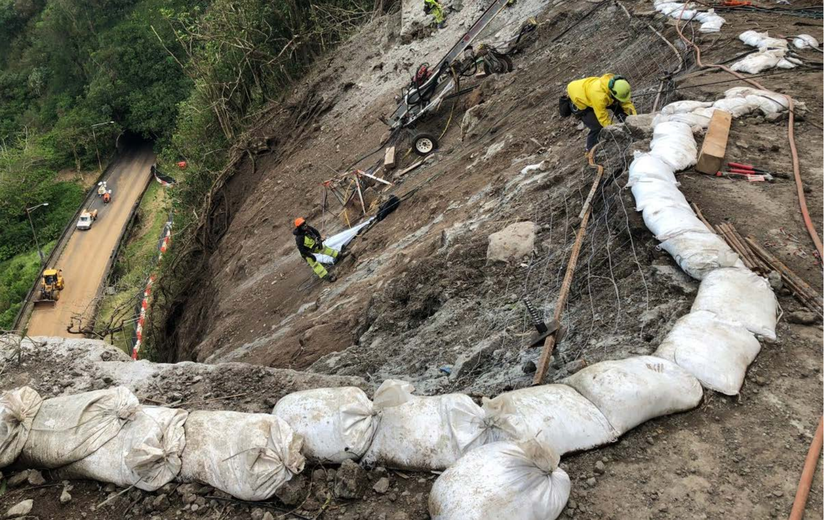
BMPs are implemented during rockfall mitigation off Pali Highway, Kaneohe, Hawaii.
