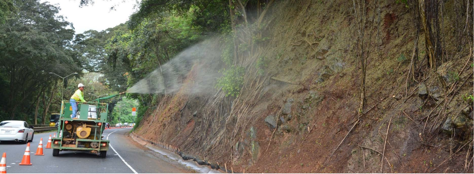
High performance erosion control mulch is used to stabilize significant erosional areas along Kalanianaʻole Highway, Kailua.
