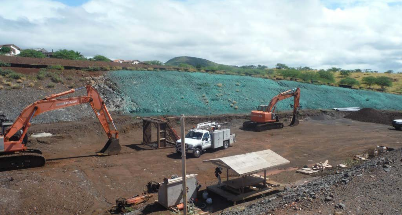
Construction BMPs are implemented on the Kapolei Interchange Complex construction project.
