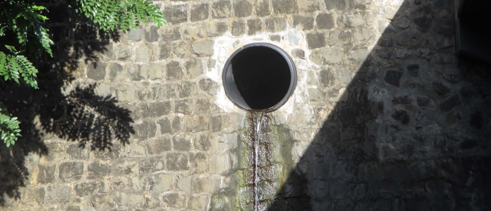
Inspectors monitor outfalls for illicit discharge and pollutants.
