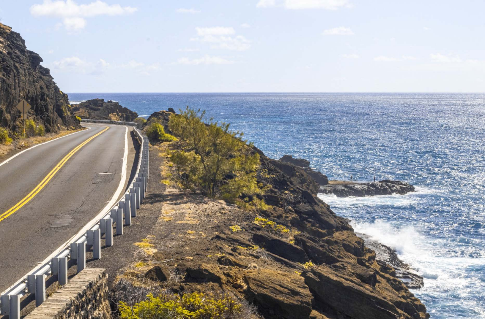
DOT-HWYS maintains Kalanianaʻole Highway along of eastern coast of Oahu.
