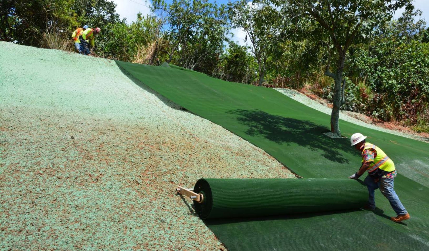
Eroded slope repair addresses sediment and nutrients loading along Kalanianaʻole Highway in Kailua, Hawaii.
