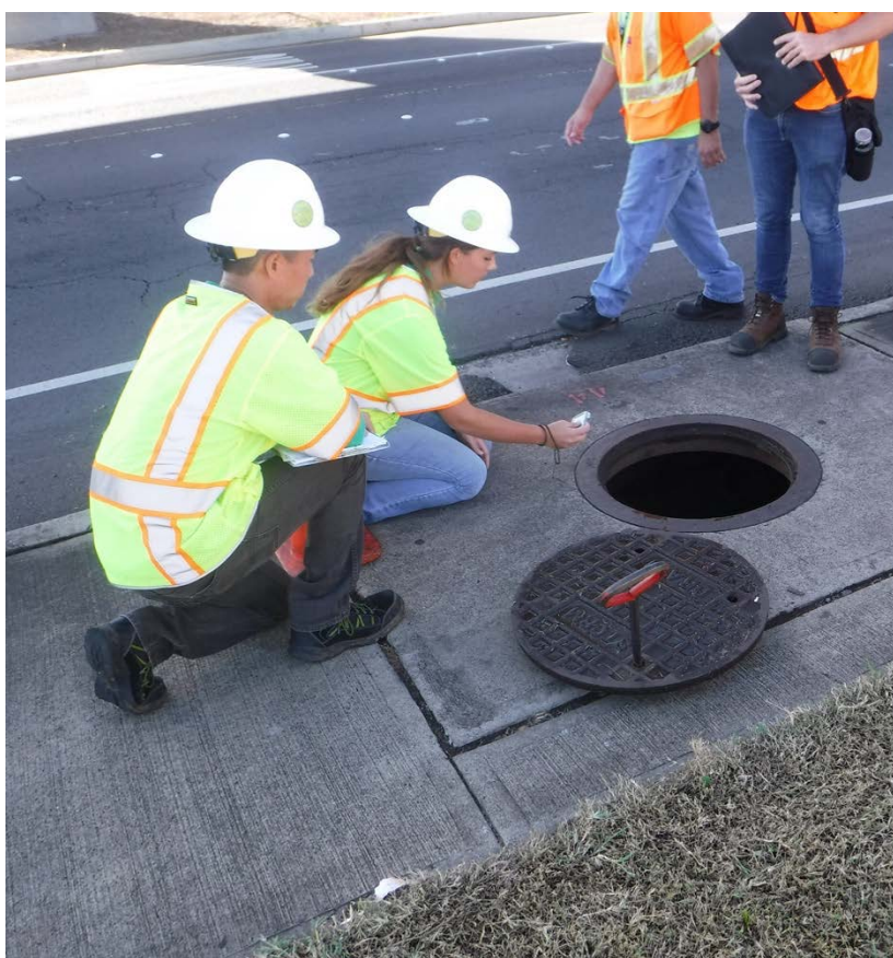
A team of inspectors document a connection.
