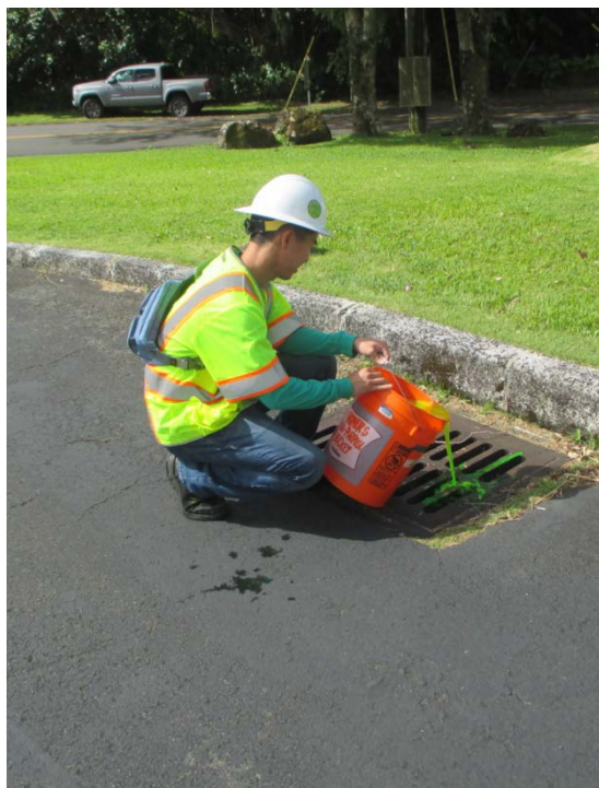
An inspector performs a dye test to verify the connectivity of the private drainage structure to the DOT-HWYS MS4.
