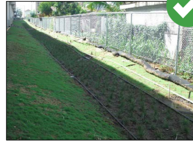
Additional watering or irrigation to supplement rainfall may be needed until vegetation has been established.
