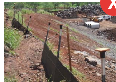
Avoid using silt fences on slopes. However, if silt fence is placed on a slope, the fence post may need additional embedment.
