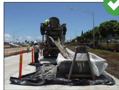
Concrete washout area must be lined with an impermeable material. Secondary containment under washout catches any leaks or splashes from the washout area.
