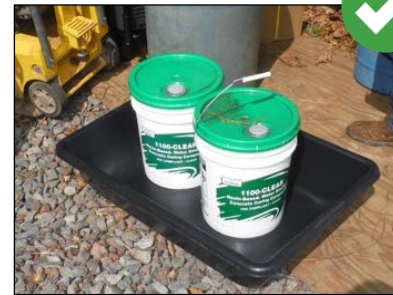
Secondary containment reduces the risk of spills and leaks from getting into storm water runoff, contaminating soil, and injuring workers or visitors.
