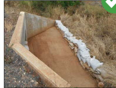
Sandbags may be stacked in a brick wall-like formation if additional reinforcement is used.
