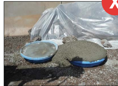
Concrete washouts must be changed or not used after reaching 75% capacity or 4-inch freeboard, whichever is more stringent. Hardened concrete should be removed frequently to avoid overcapacity of washout area.
