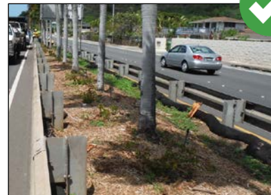
Evenly distribute wood/bark chips on soil surface and maintain a 2-inch mulch depth to tree basins and a 4-inch mulch depth to shrub beds.
