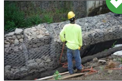
Gabions must be filled with a well graded mixture of aggregate, with larger stones being predominant and smaller stones to fill the voids.
