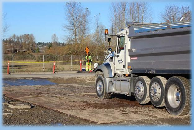
Rock construction entrances cost between \$6,500-\$8,000 from installation to disposal in landfill. Metal and plastic entrances cost between \$8,000-\$10,000 one time and are 100% reusable.
