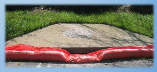
Device works well in small rain events. Prone to flooding in large events and can clog without frequent maintenance. 50% reusable.
