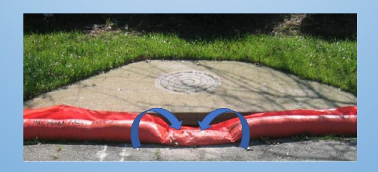
The best BMP device has overflow capability to reduce any chance of clogging/flooding
