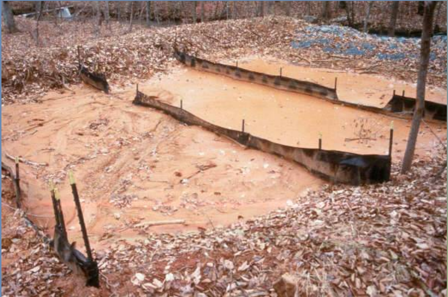
Sediment Trap with Baffles
