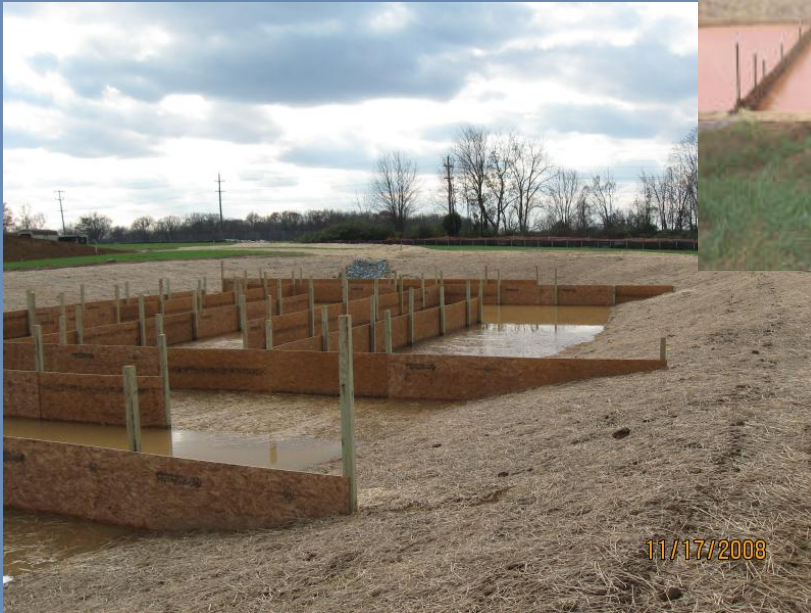
Baffles in sediment Basins
