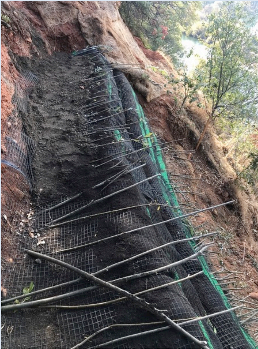
Biaxial Geogrid added for structural reinforcement
