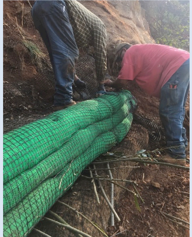
Gripple Anchor System used to tieback geogrid to slope - 500 lbs. working strength
